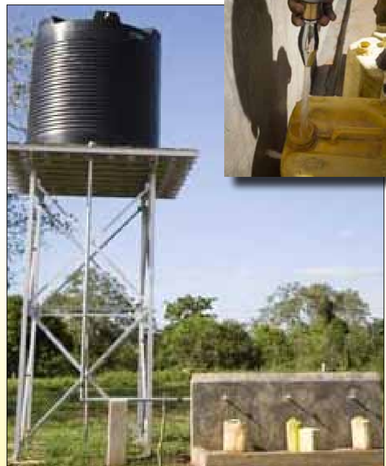
A typical 3-point water supply, Kamuli District Inset: A self-closing water tap prevents wastage
