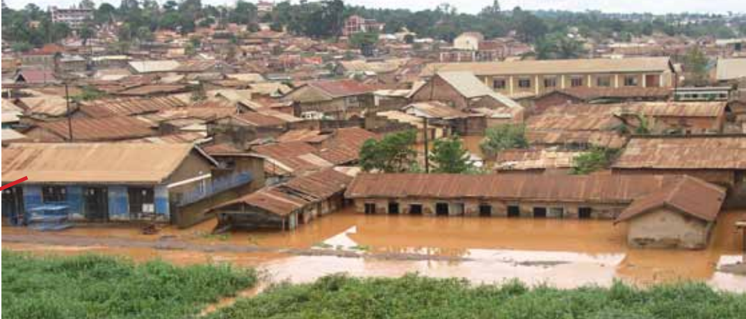
Flooding in Nsooba Lubigi drainage channel. Houses and a school are submerged in the water in 2007.
