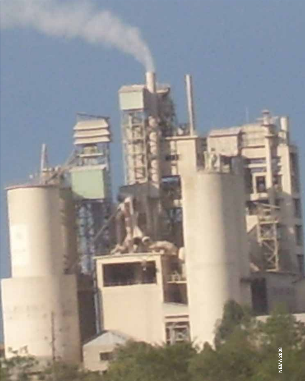
Hima Cement Factory, Kasese District in Western Uganda (2008)
