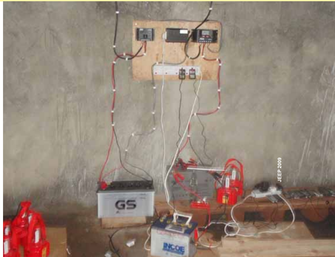
Solar power: Phone, battery and lantern charging in rural Wobutungulu by a solar project implemented by Joint Energy and Environment Projects (JEEP), a local NGO.
