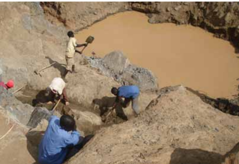
Construction of Nyagak Hydro electric power plant
