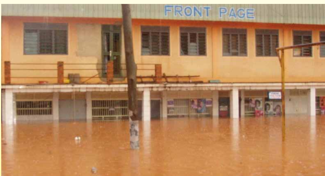
These buildings were constructed in wetlands which are the water ways for drainage into Lake Victoria. The houses were flooded in 2007 temporarily interfering with traffic and business along the Kampala-Entebbe highway.
