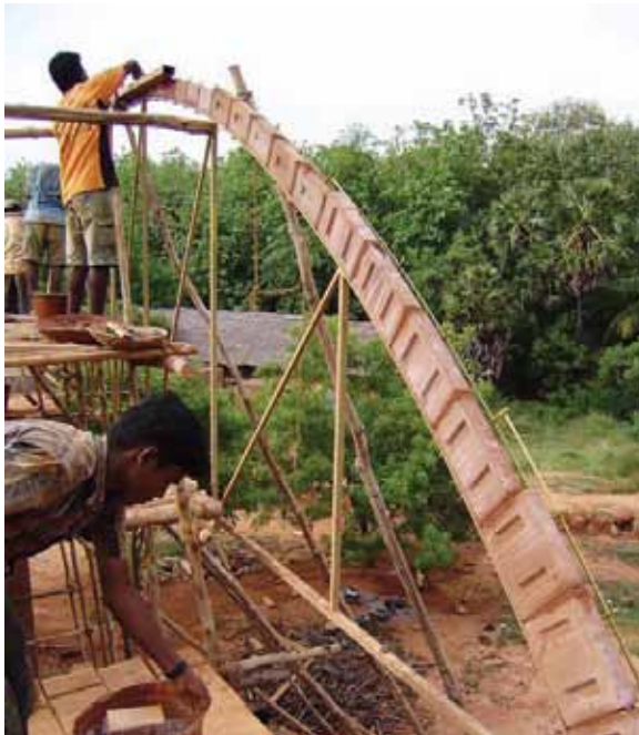
Figure 5: Precision being executed at site
