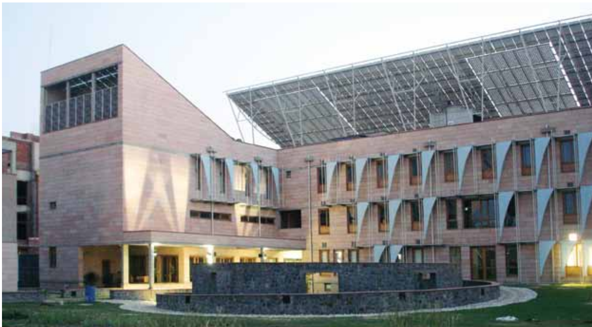
Figure 19: PV panels shading the roof
