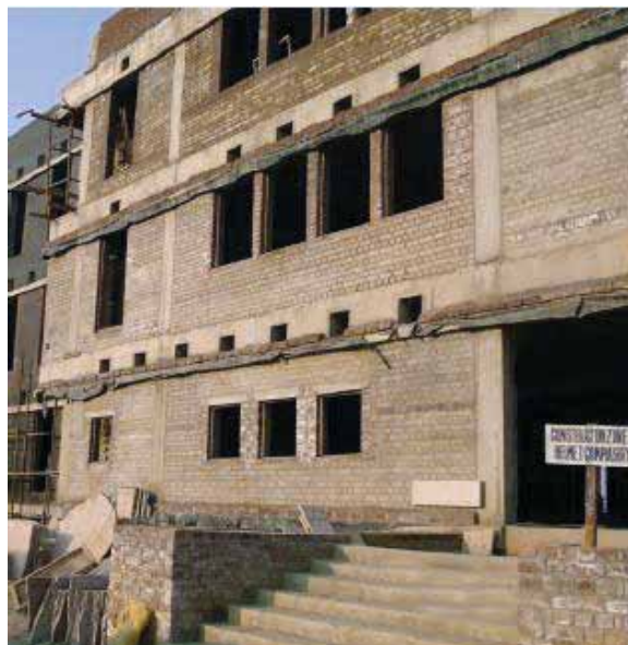
Figure 16: Compressed Earth Block instead of burnt brick
