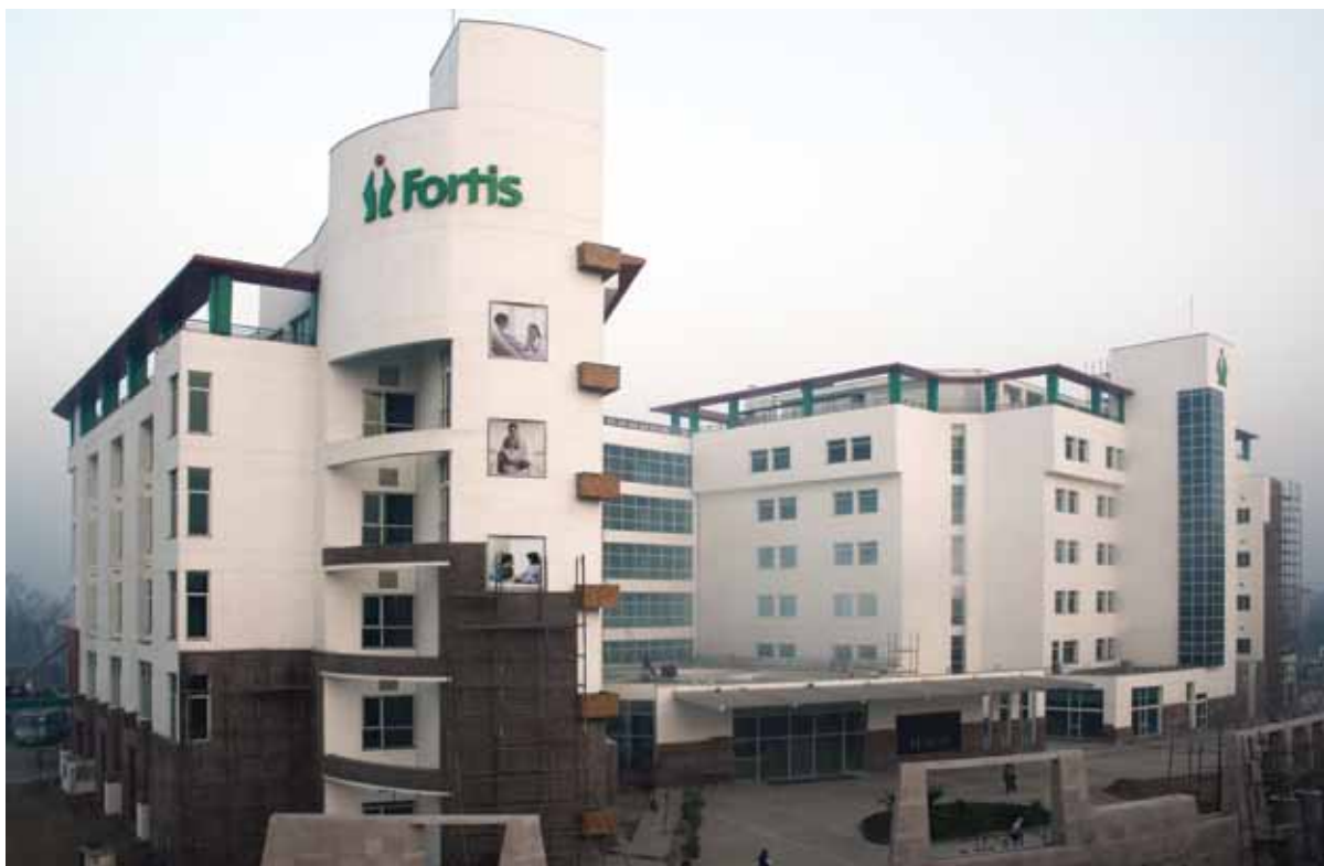
Figure 20: Image of the ECBC compliant Fortis hospital building at Shalimar Bagh
