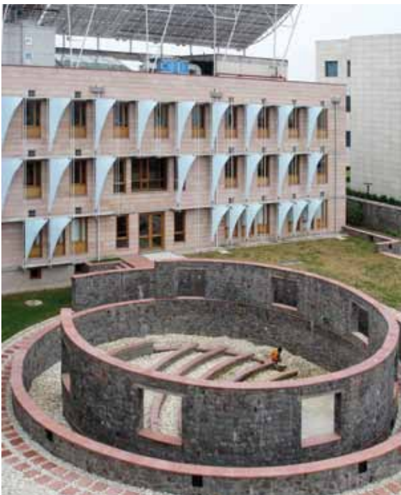
Figure 15: Amphitheatre acts as the filter bed for with rainwater storage tank below it
