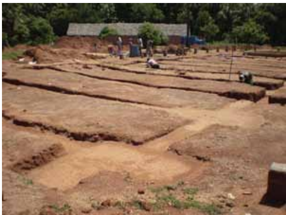
Figure 4: Rammed foundations
