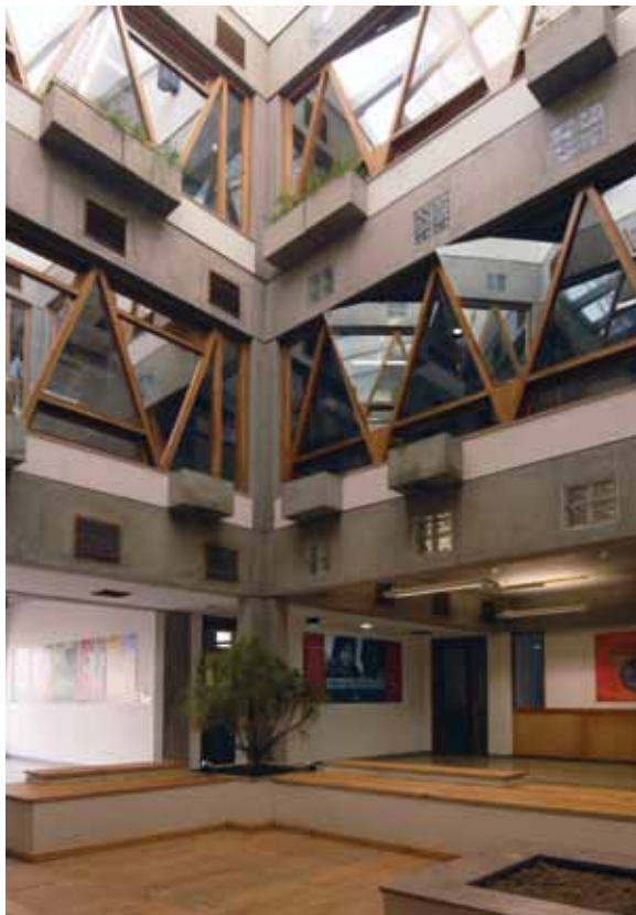
Figure 18: Wooden air conditioning grilles instead of aluminium
