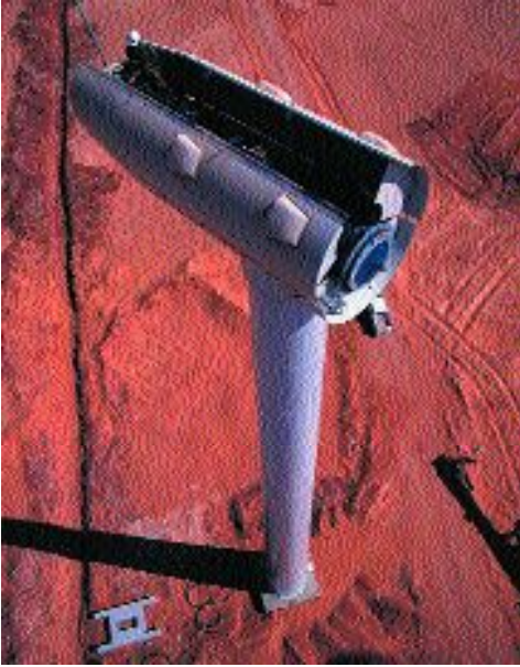
A modern grid connected wind generator being installed
