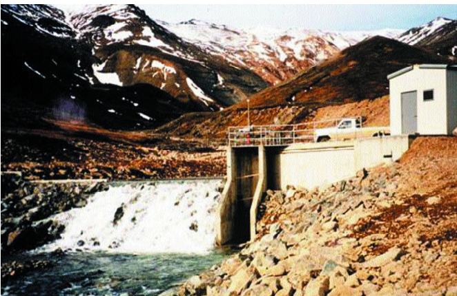
Small scale hydro system in South America (courtesy NREL)
