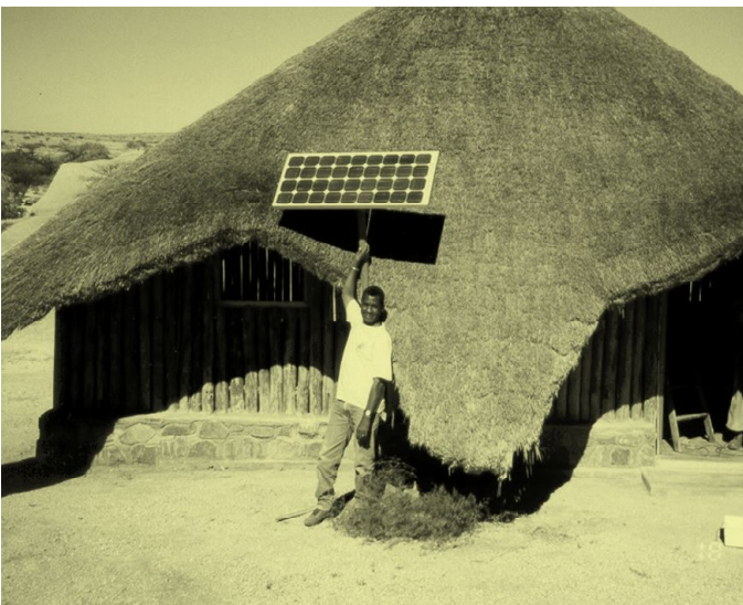
A PV module such as this one can power efficient lights for small tourist huts
