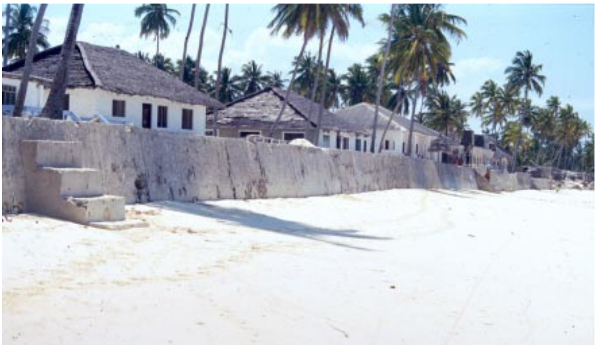
Sea wall at Jambini (Unguja)
