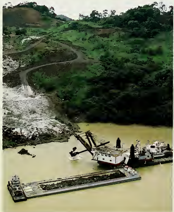
Without trees to protect the soil landslides are common.
