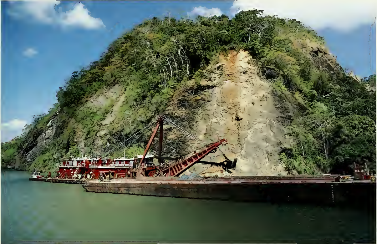
Continuous dredging is necessary to keep the canal open.
