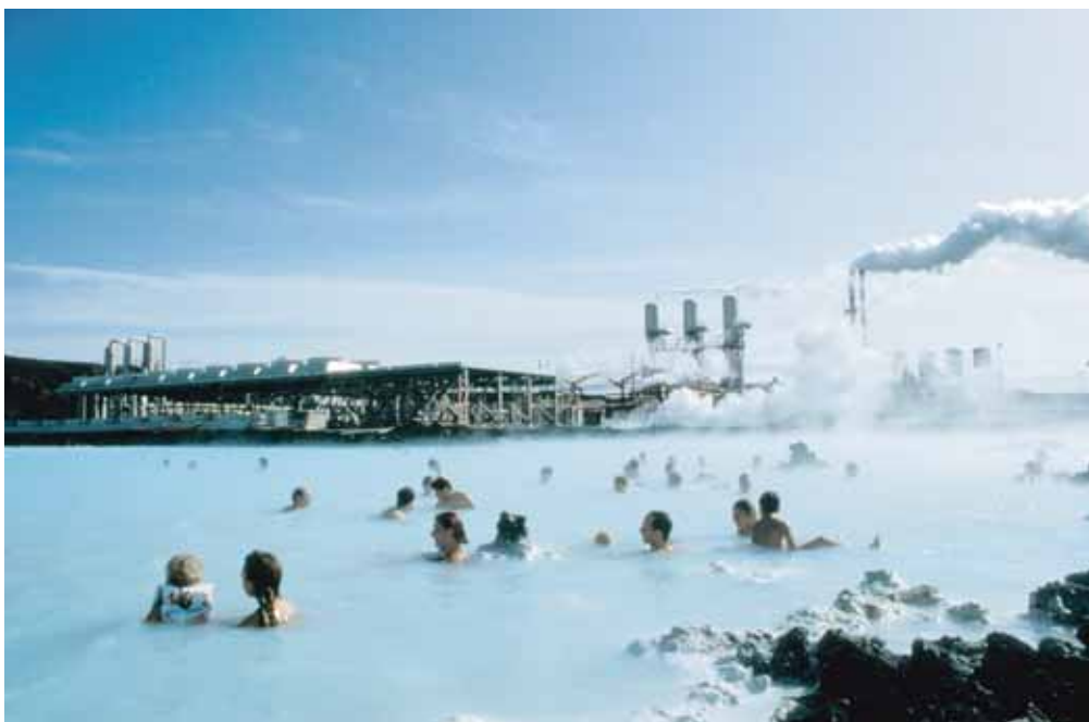
Geothermal power plant, Iceland.
