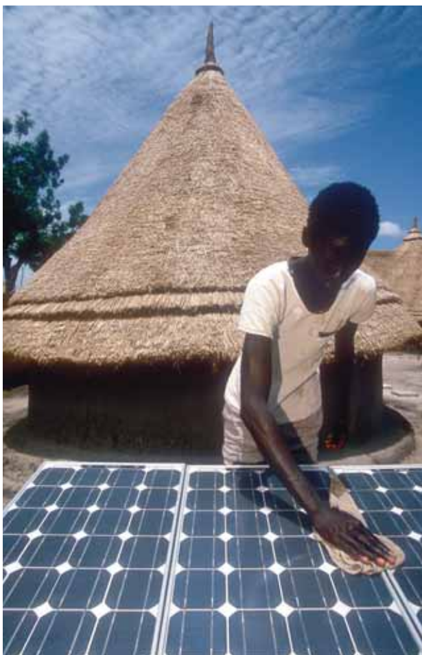
Solar and wind energy are promising options for rural areas that are not connected to the electricity supply grid.
