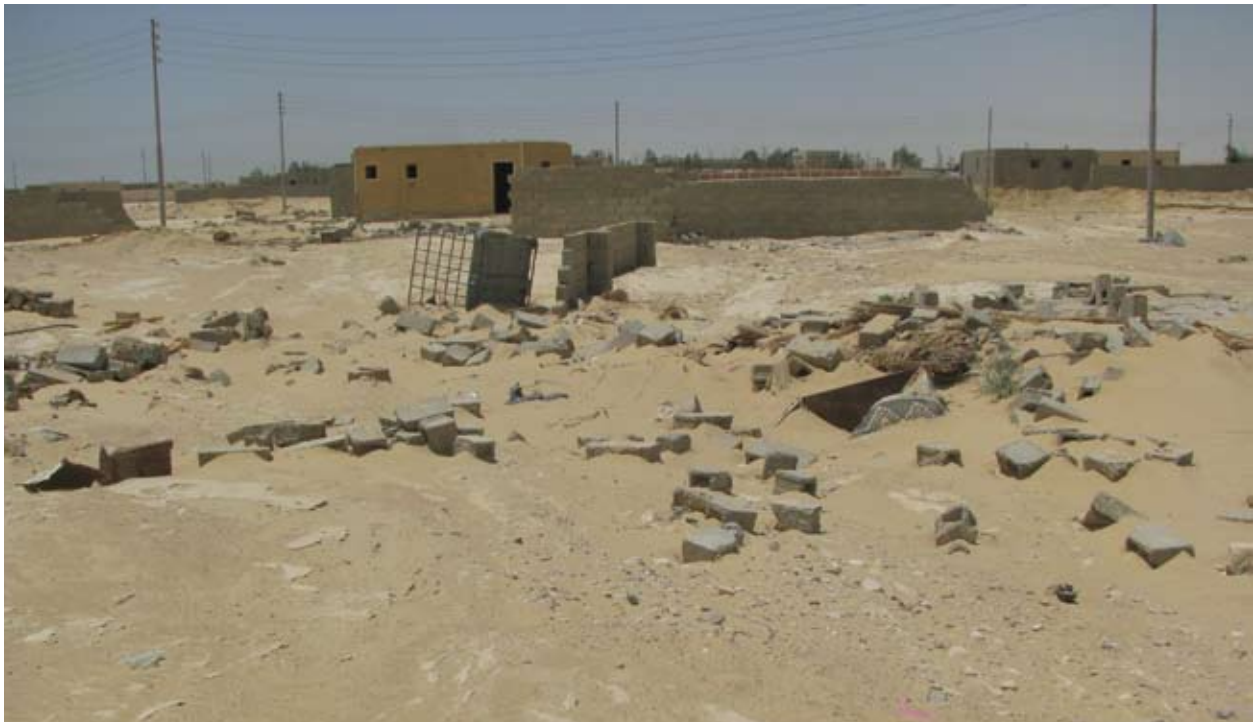
Impact of Recent Flashflood on Bedouin Houses
