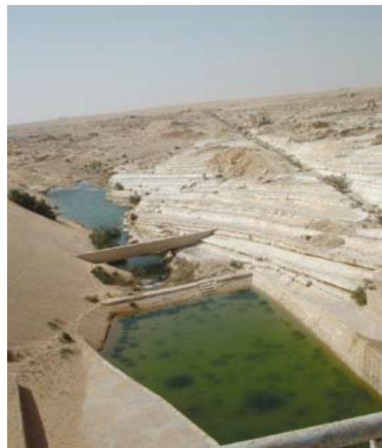
A government built dam to collect flashflood water around the assessment area
