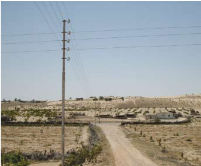
Clean and well maintained roads are basic requirements for communities to develop
