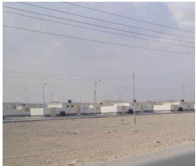
New houses built by the government for Bedouin in El Hassana Source: Mohamed Tawfic
