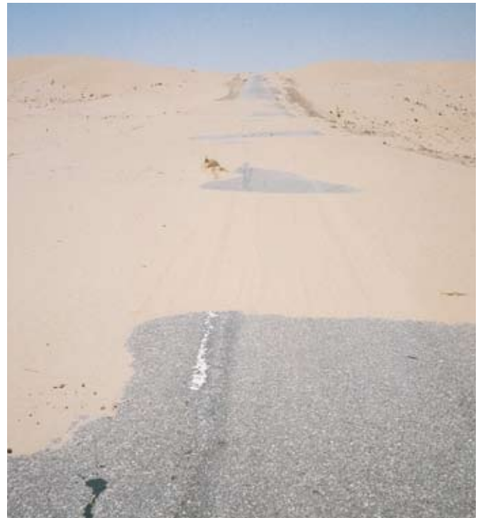
The main road of El Maghara area covered with sand Source: Mohamed Tawfic
