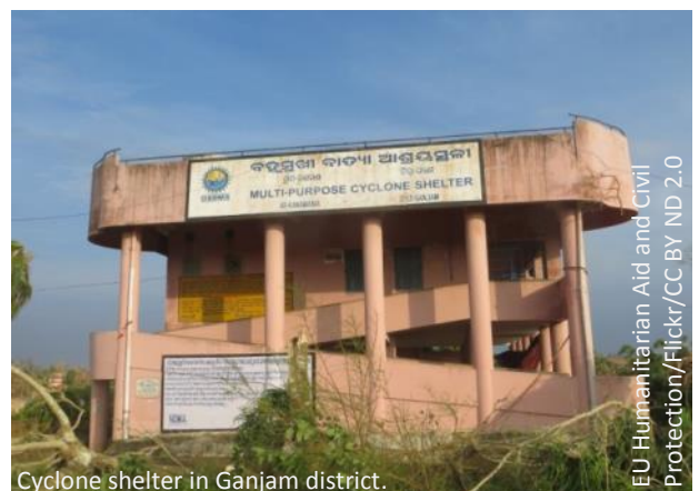
Cyclone shelter in Ganjam district.
