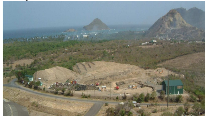
Figure 2-13 Vieux Fort Solid Waste Management Facility
