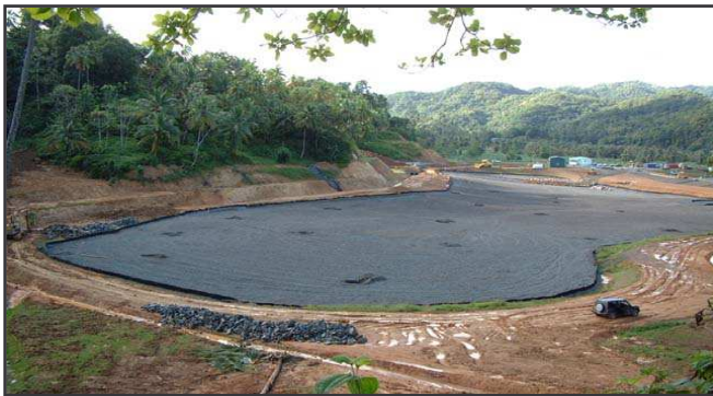
Figure 2-12 Deglos Sanitary Landfill
