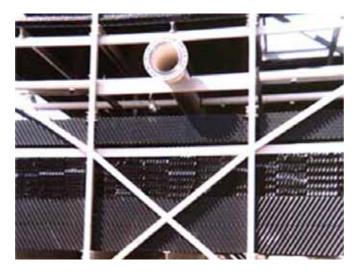
Figure 6 Water spraying frame and contact buffer
