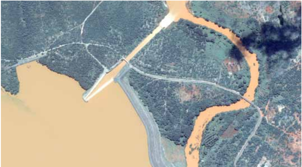
Google Earth image of the outflow of the Masinga Dam and the Masinga Power Station, on the Tana River, in November 2003, during the short rainy season
