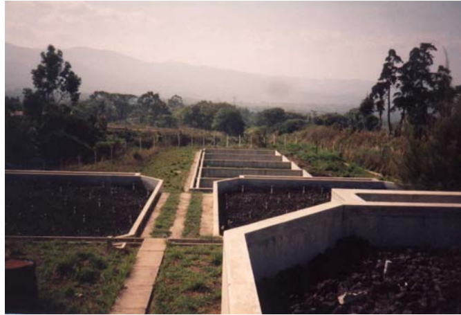
Low technology version of a clarifier. Imhold tank provides primary sedimentation at the plant.
