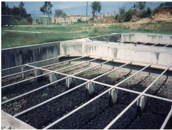
Low technology version of a clarifier. Imhold tank provides primary sedimentation at the plant.
