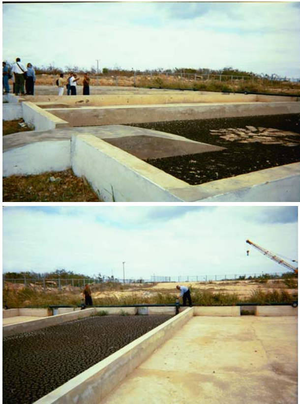
Activated sludge being wasted to drying beds. Dried sludge on concrete drying beds.
