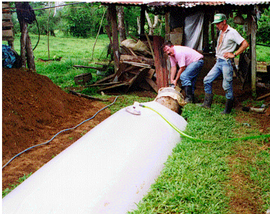
Installation of biodigestor.
