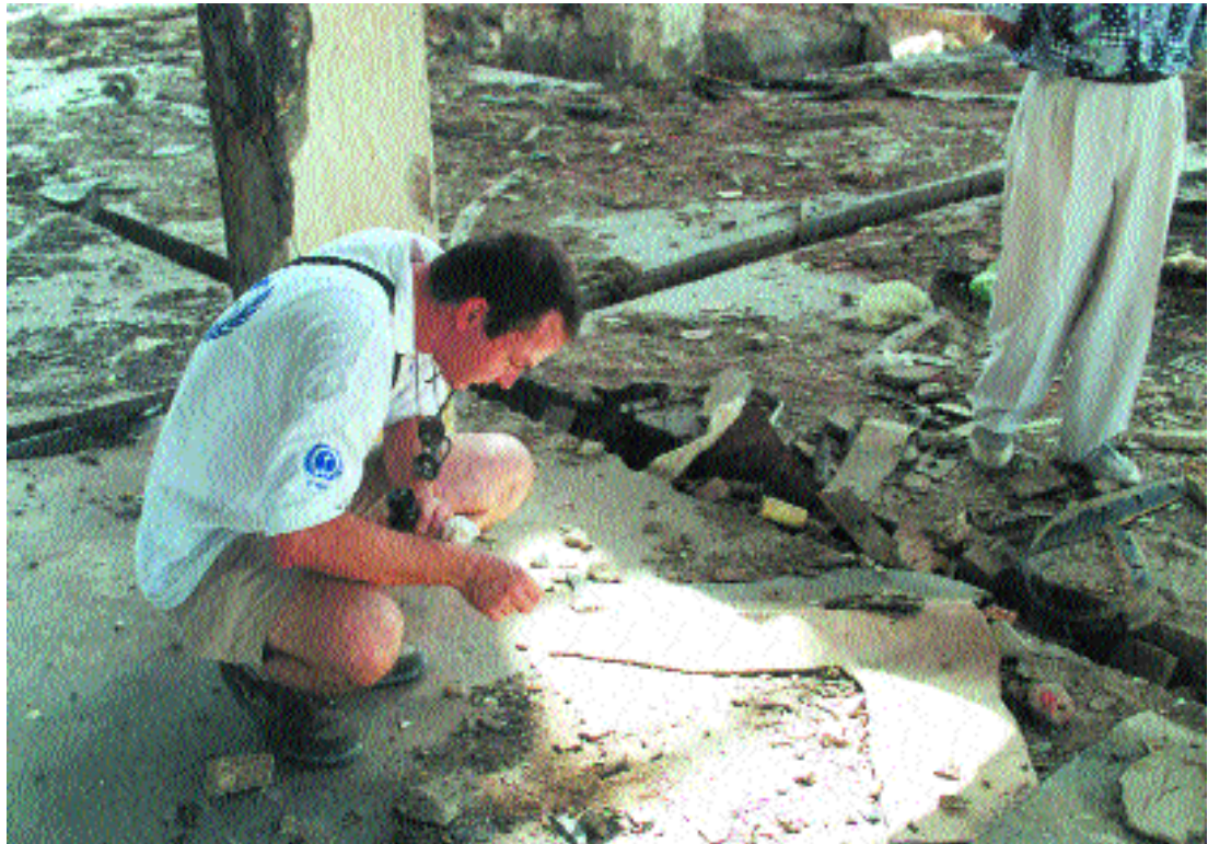
Site inspection at Vlorë complex
