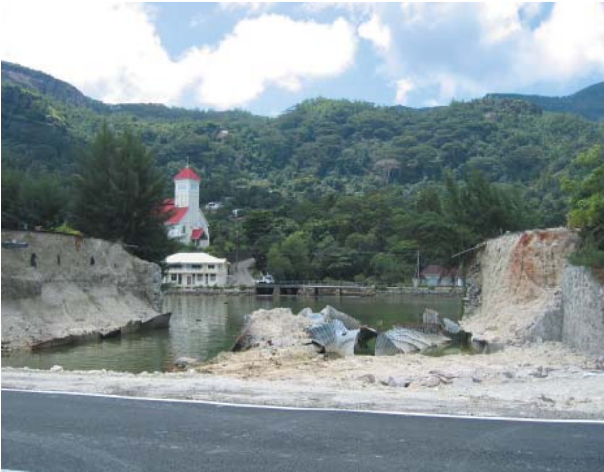
The remains of a road swept away by the tsunami (photo taken from repaired section). Credit: M. de Vries
