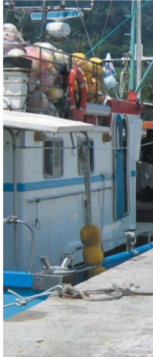
Peer damage caused by the tsunami storm surge. Credit: M. de Vries
