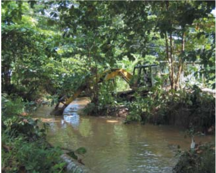
Dredging a clogged discharge channel. Credit: M. de Vries
