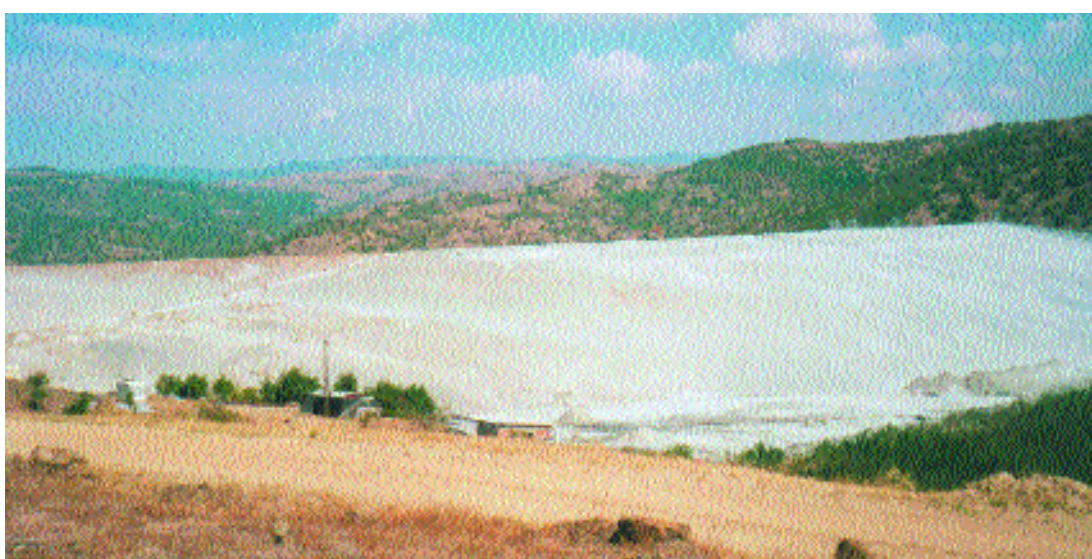
Hydro-tailing dam near Buchim S.C. mine
