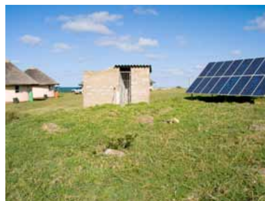
Increased use of solar energy would reduce indoor air pollution
