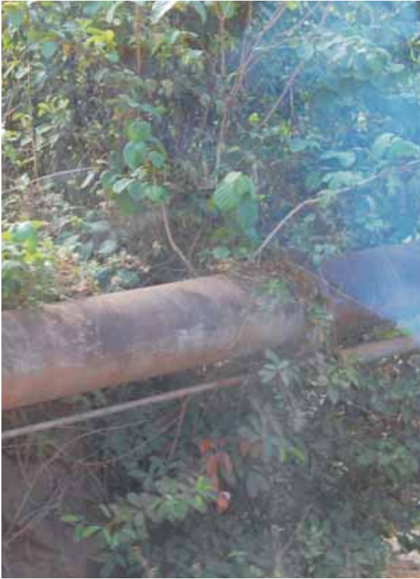
The main municipal water pipe for Freetown carries fresh water from dams in the Western Area catchment, but can only serve a limited portion of the population
