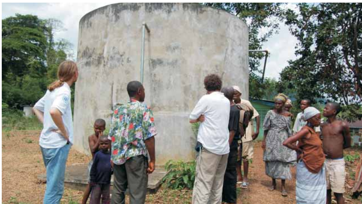
This concrete silo was one of the few things to survive an RUF attack in rural Kenema District. Most of the other water infrastructure in the region was damaged or destroyed
