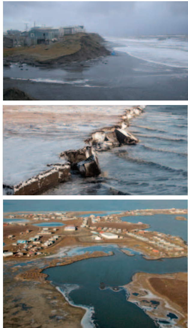
Figure 9.40. Beach erosion at Ukkuqsi, Barrow Alaska (upper). Photo courtesy of Anne Jensen. Erosion at Tuktoyaktuk, Northwest Territories, Canada (middle). The shore has eroded as much as 200 m in 55 years in some locations. Concrete and rock revetments now protect parts of the outer coast (lower), but erosion continues at the unprotected locations. Erosion of the uninhabited and unprotected island at the harbor mouth will threaten the long-term viability of the harbor within the next 50 years. Middle and lower photos: Martin Fortier/ArcticNet.
