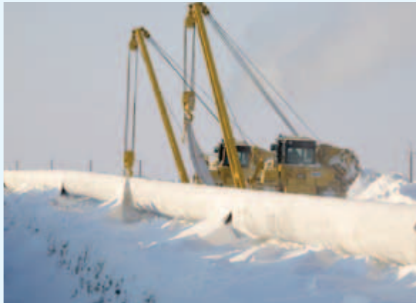
Figure 10.5. Pipeline under construction in the Russian Arctic.
