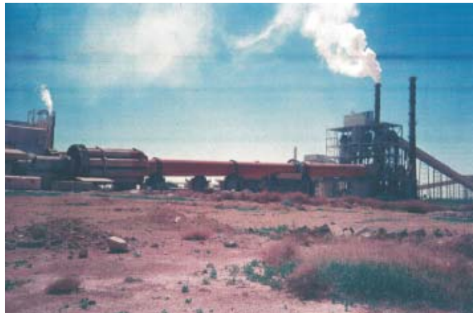
A cement factory in Iraq
