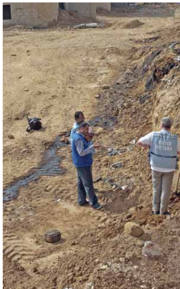
Landfill leachate leaking from Rafah landfill
