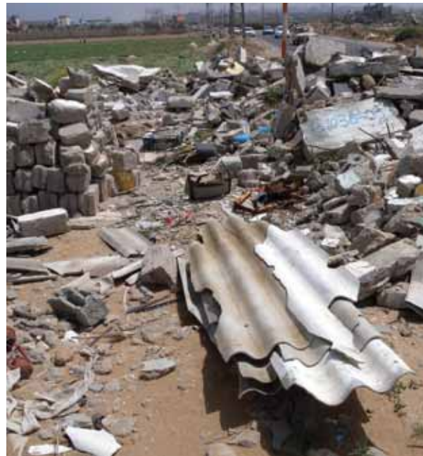
Asbestos in rubble
