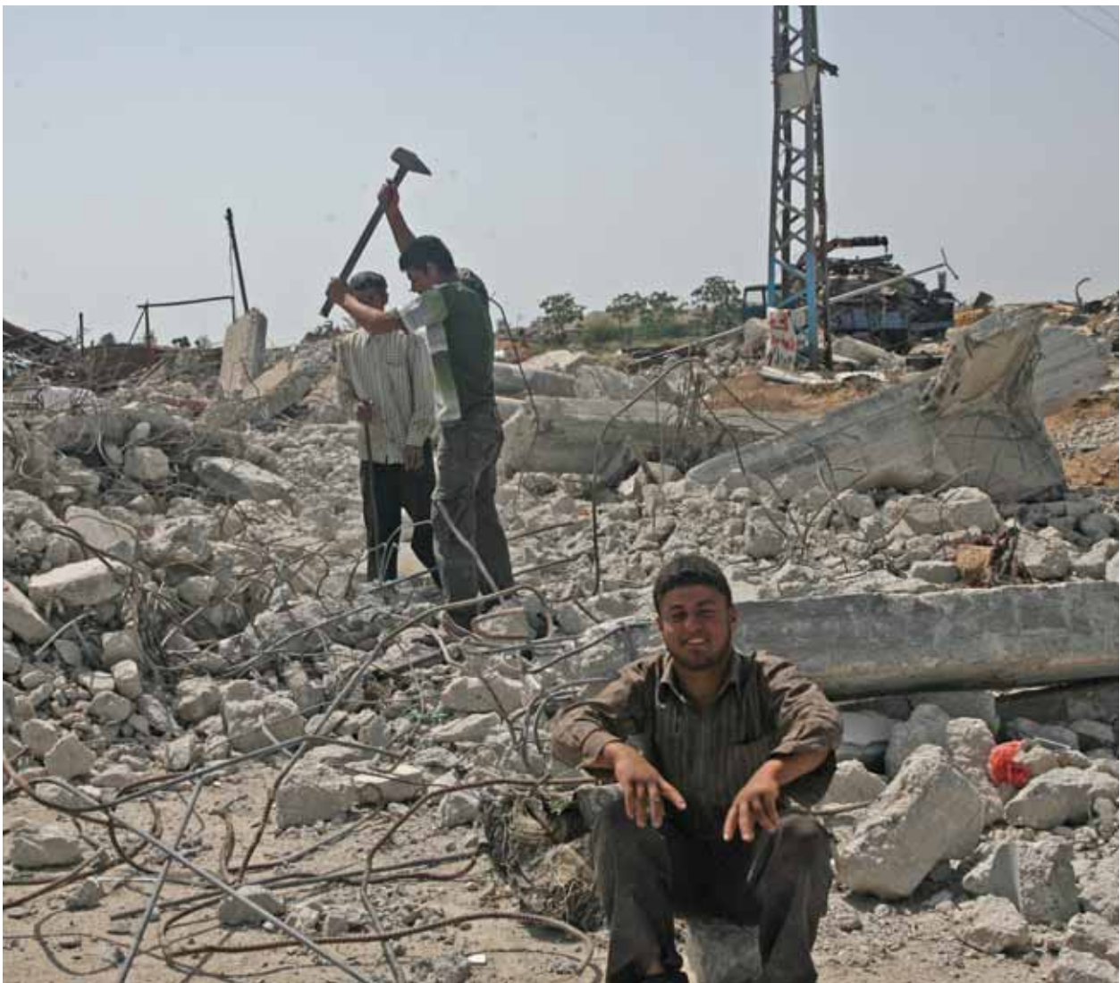
Workers recovering reinforcement bars from the rubble
