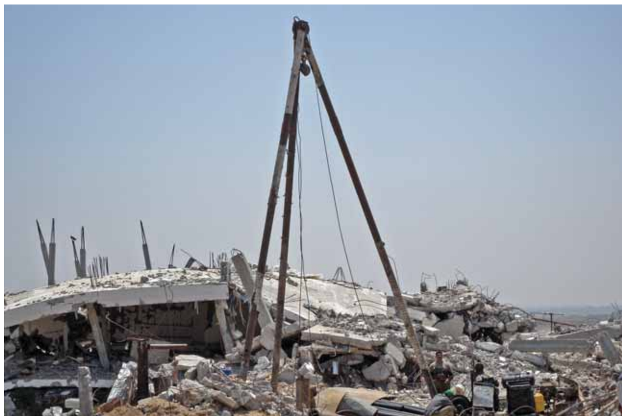
Private well drilling operation in northern Gaza Strip
