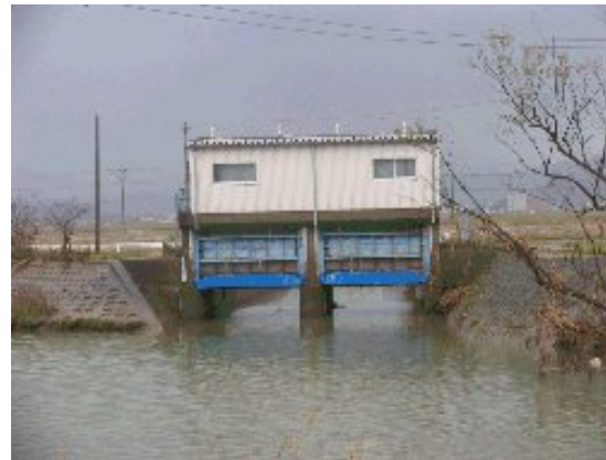
Maruyama River's sluice pump system
