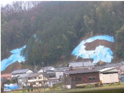
Landslide sites covered by plastic sheeting
