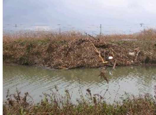
Extensive forest debris along river banks
