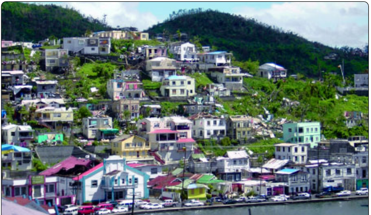
Hurricane damage in Grenada
