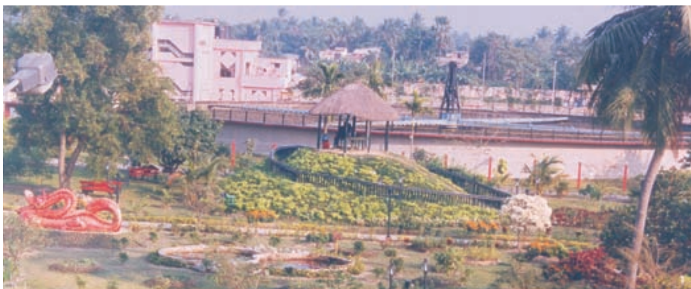
Sewage Treatment Plant with attractive surroundings at Chandan Nagar in West Bengal
