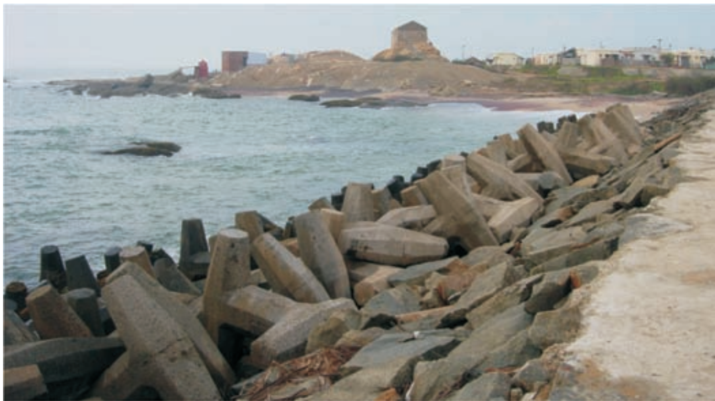
Prevention of coastal erosion at Kanya Kumari
