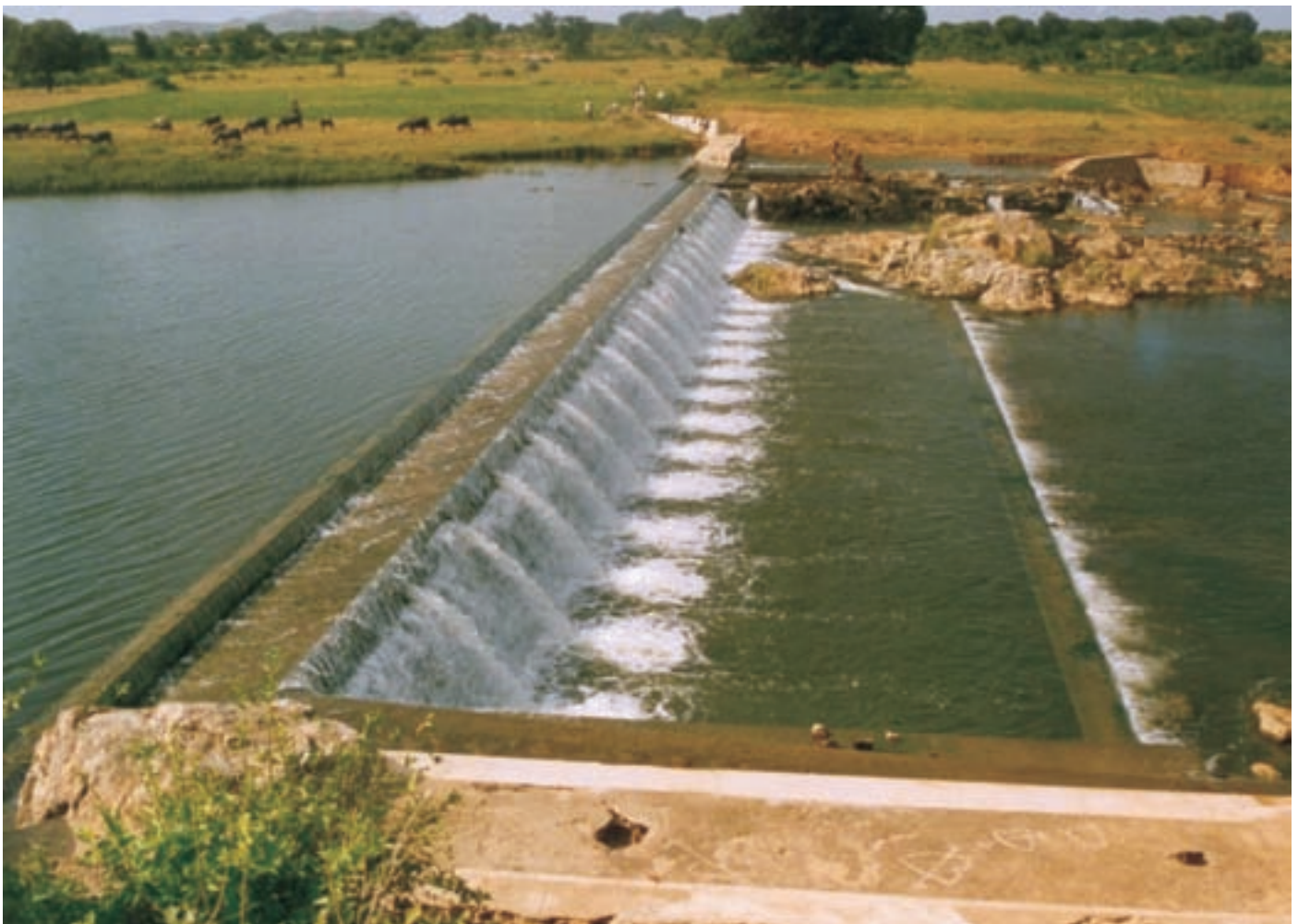
Check dam in Bundelkhand : Small is sustainable
