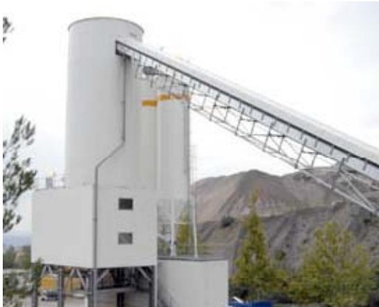
Example of a concrete-mixing plant.
