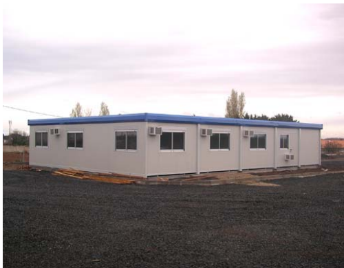
Example of site living quarters (unit model)
