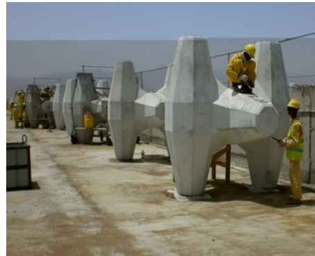
Top left: view of the CORE-LOC™ artificial rockfill
