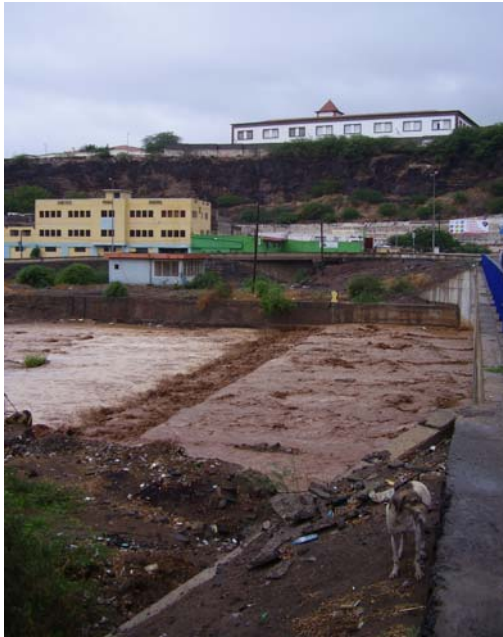
Storms of 29 August 2007: flood in the Ribeira de Trindade (Trindade River) around the main bridge.
