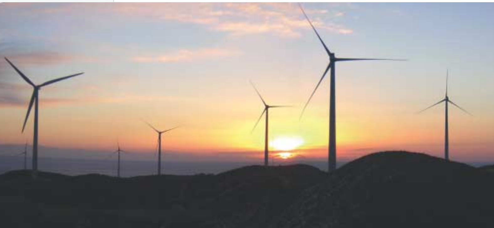
Yeongdeok Wind Power Plant, Gyeongsangbuk-do
