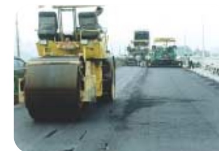
Asphalting a road with recycled aggregates
