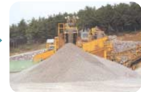
Construction wastes shredded into minute pieces
