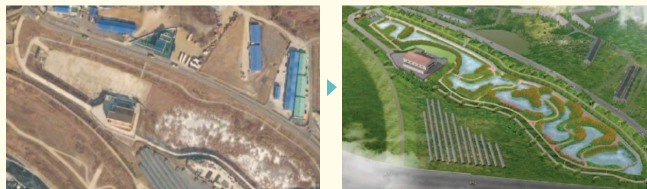
● Rain Water Pumping Station – Before Restoration ● Rain Water Pumping Station – After Restoration
