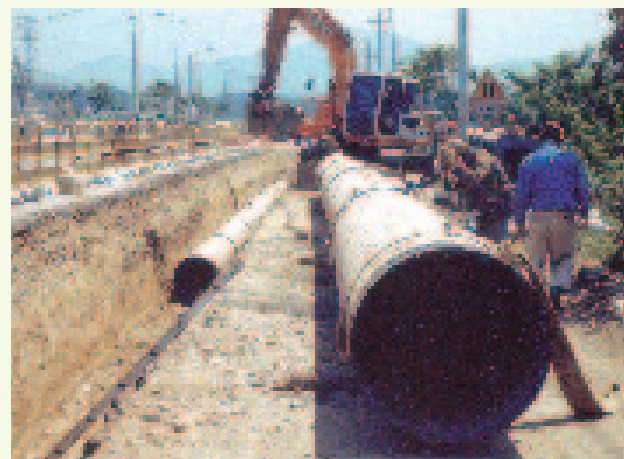
Replacing Aged Water Pipelines
