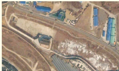
● Rain Water Pumping Station – Before Restoration
