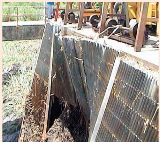
Siltation greatly reduces the capacity of hydroelectric generators in Malawi. It collects in grates and filters, necessitating constant maintenance, and damages turbines. A functioning intake filter is seen below left, while one damaged by silt and debris can be seen on right.
