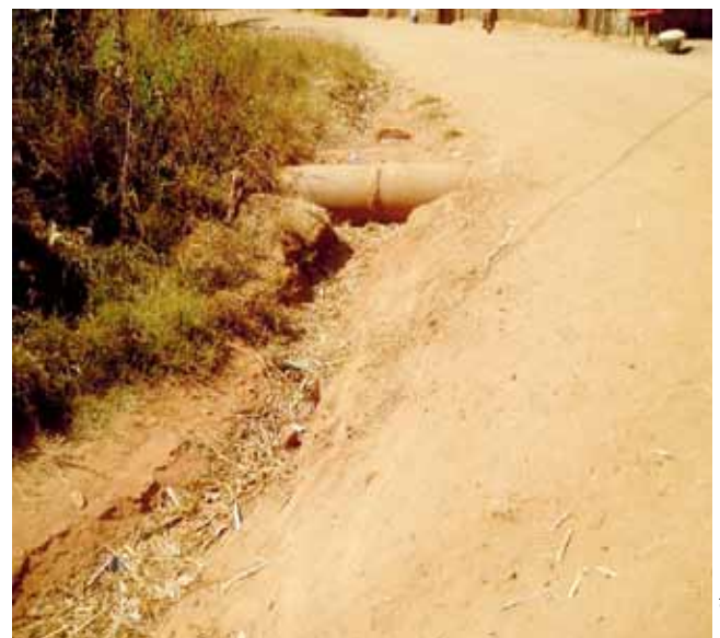
Erosion of road drains.
