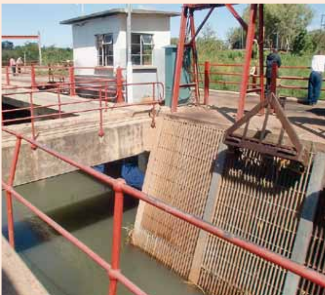
Siltation greatly reduces the capacity of hydroelectric generators in Malawi. It collects in grates and filters, necessitating constant maintenance, and damages turbines. A functioning intake filter is seen below left, while one damaged by silt and debris can be seen on right.
