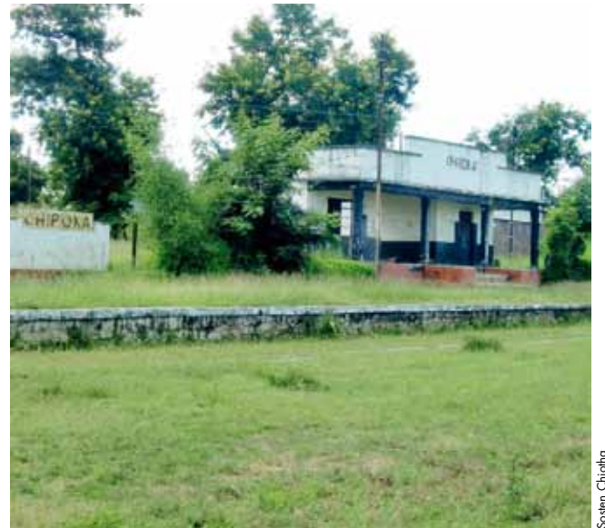
Rail transportation is inexpensive and can ease the pressure from road networks. Restoration of existing railway networks (e.g. Chipoka Railway Station shown in photo) will help to achieve this.
