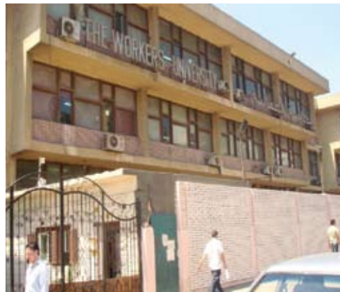
Picture (4-3) Noise Monitoring Terminal located in Workers University- Autostrad road
