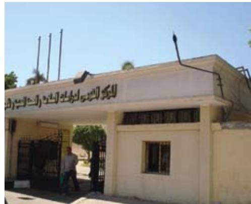
Picture (4-6) Noise Monitoring Terminal located at the Occupational Safety National Center – El Hegaz Street
