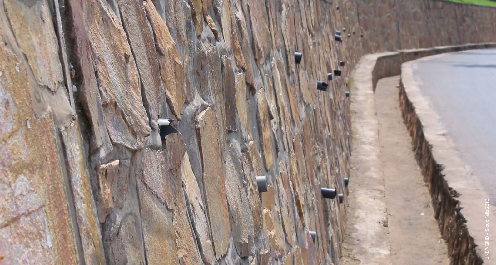
Some streets in Kigali are lined with open drainage canals and vented retaining walls to help channel runoff and rainwater
