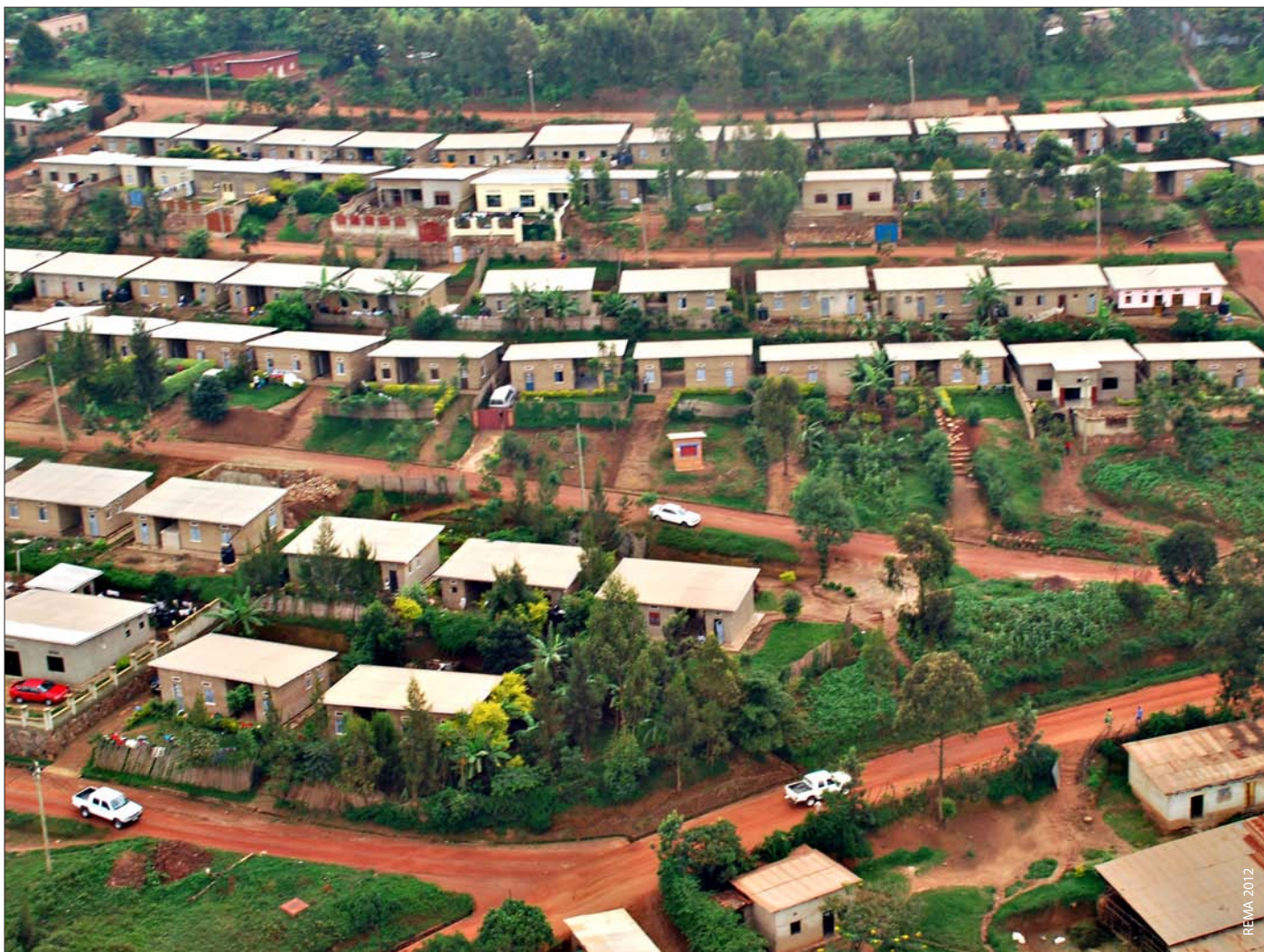
Earthen brick houses line the streets of Batsinda
