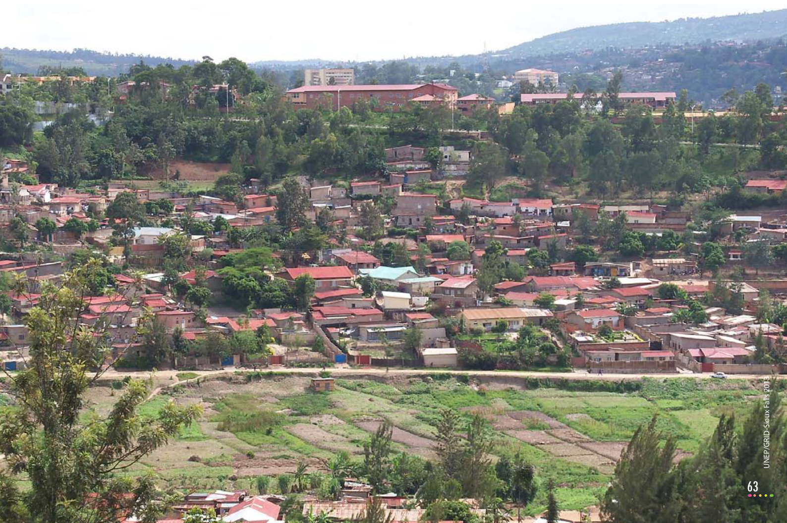
Houses built on a hillside in Kimihurura across from the Kacyiru wetland
