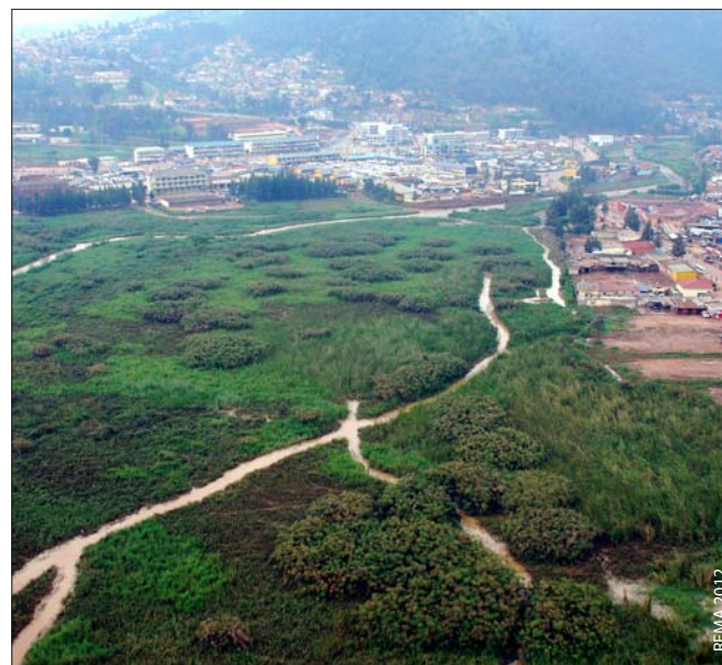
Flooding is problematic in Gatsata because there are many input rivers and tributaries, but only one output — the Nyabugogo River
