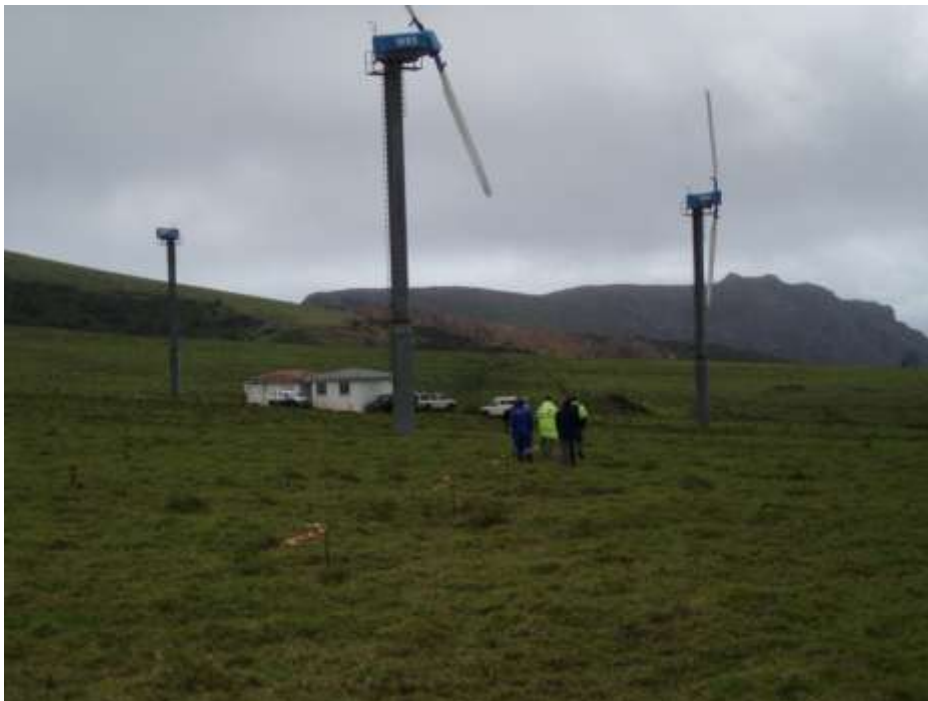
Figure 6.1.1 Wind turbines at Deadwood Plain - EMD
