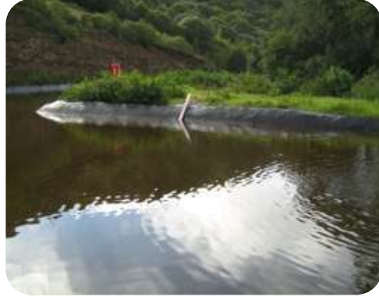
Plate 2.1: Scotts Mill Reservoir which supplies the Red Hill distribution area. © Connect St Helena Ltd., 2013.
