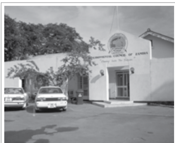
Environmental Council of Zambia Offices in -Lusaka
