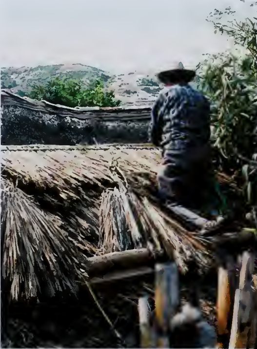
Re-thatching a roof with the versatile soyate palm in the community of Topiltepec, Guerrero, Mexico.
