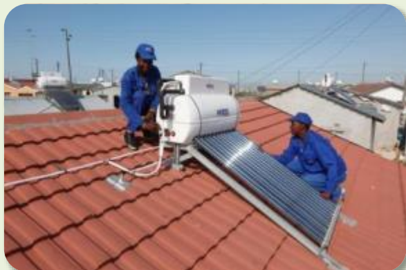
Installation of solar water heaters on houses as part of the Kuyasa project, South Africa. Photos: Nic Bothma
