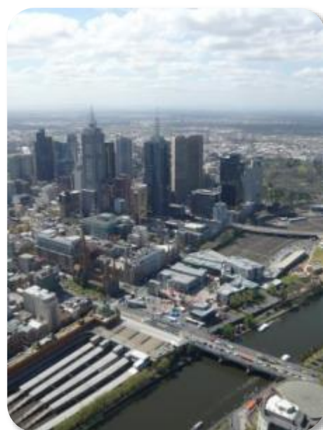
Melbourne, Australia is engaging with the cCCR, with actions including a programme for energy efficiency for buildings and a 'Carbon Neutral Council'. Photo: ENERGIES 2050
