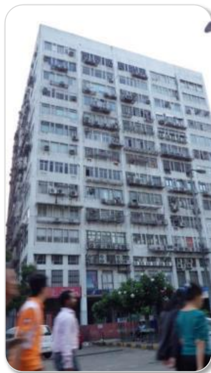
The GHG inventory for New Delhi, India reported on the cCCR shows the residential sector accounts for a third of all emissions. Photo: ENERGIES 2050
