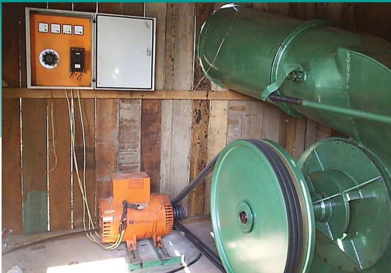
Micro-hydropower turbine and generator, part of a pilot project to install a renewable-energy "mini-grid" for the remote village of Cachoeira do Aruã in Brazil, 145 km from Santarém up a tributary of the Amazon. Photo credit: Indalma Industria/Nazareno Natalino/USAID.
