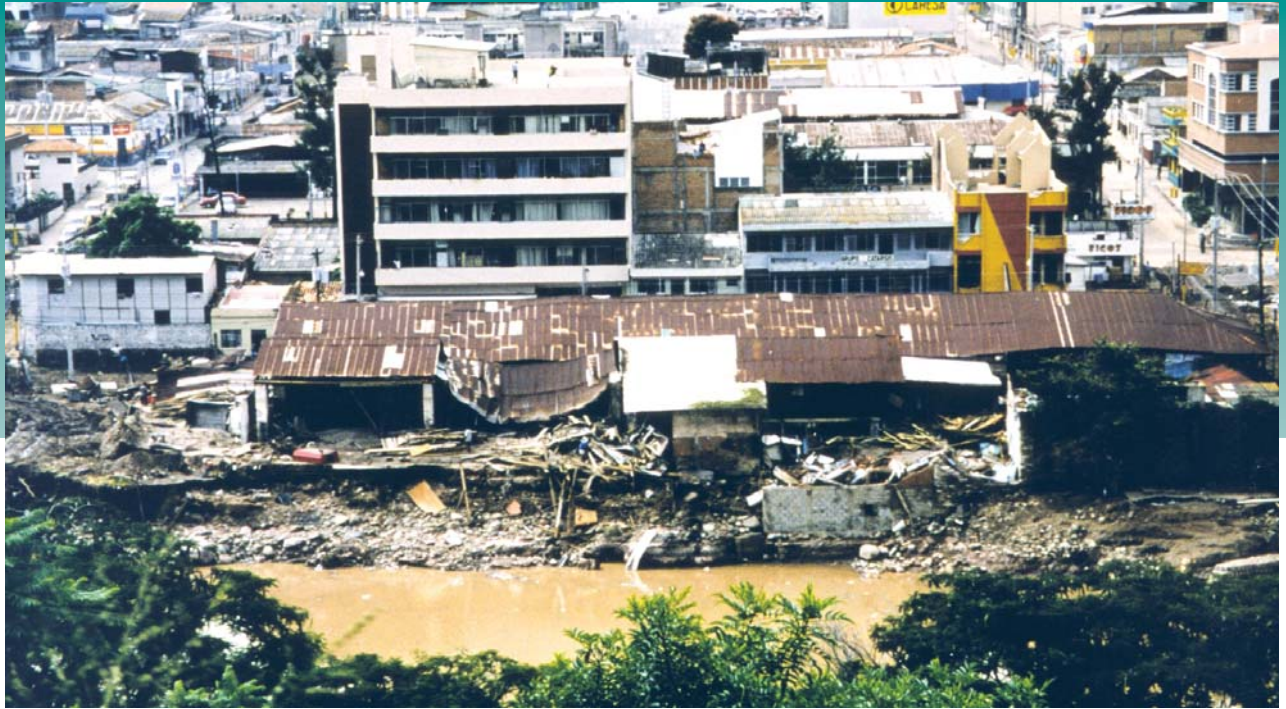
Damage along Choluteca River in the aftermath of Hurricane Mitch, Tegucigalpa, Honduras. Photo credit: Debbie Larson, NWS, International Activities, courtesy NOAA.
