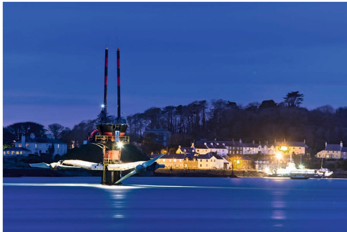
4.15 > The SeaGen tidal energy convertor in Strangford Lough in Northern Ireland is a 1.2 megawatts device whose output is comparable to that of a wind turbine. SeaGen is unusual in that it uses rotors to produce power, whereas the common method of extracting tidal energy utilizes turbines installed in a barrage wall.
