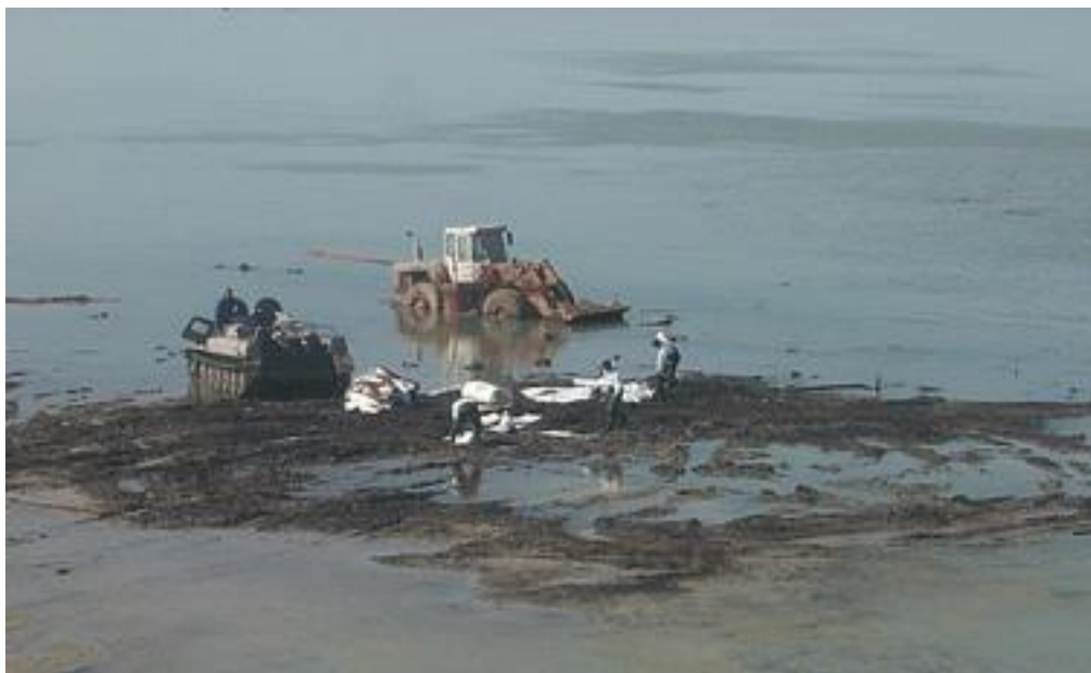
Leaks from a well at Tazhigali, oil fields, Kazakhstan
