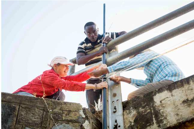
Figure 1: attaching the stilling well to a bridge over a stream.
