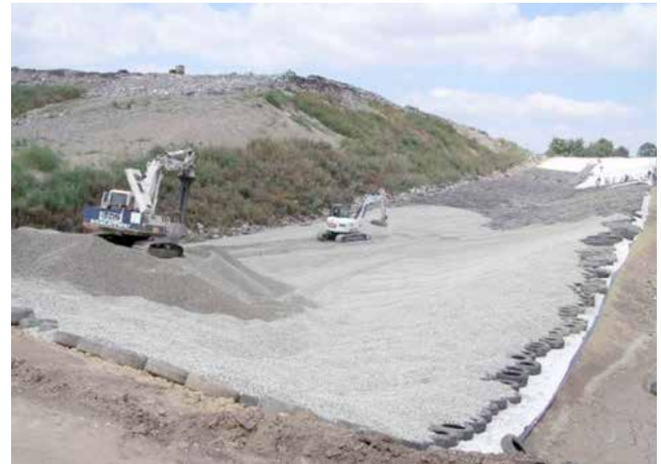
Fig. 34: Artificial geological barrier for landfill
