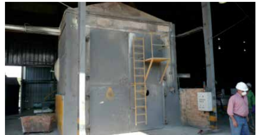
Fig. 27: Furnace of Industrias Meteoro S.A. - Dominican Republic 25 .
