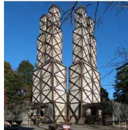
Fig. 23: Example of reverberatory furnace 28
